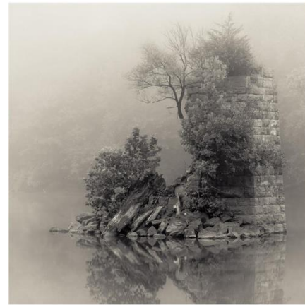
Mark Muse , Shepherdstown, WV Bridge Pier - Potomac River , 2020
